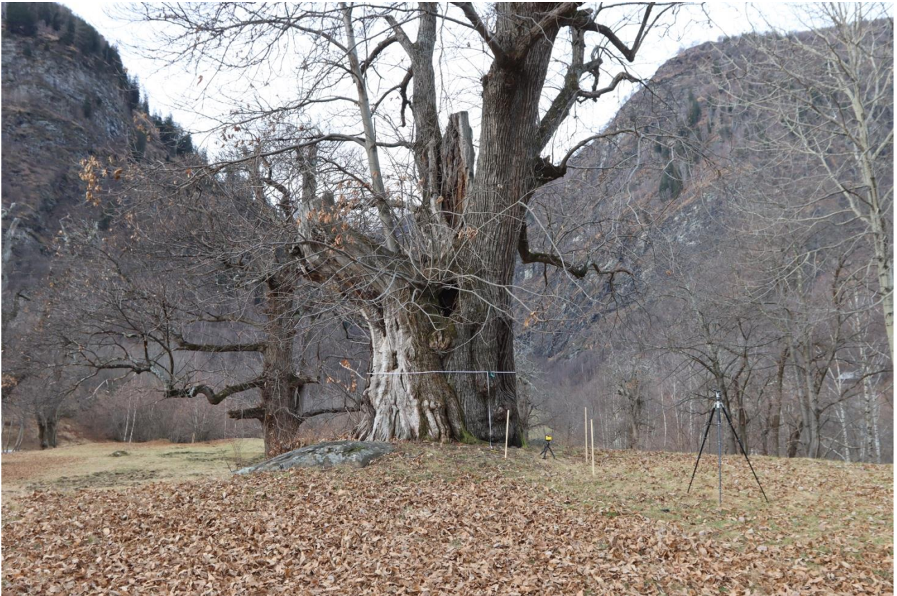
Figure 1: Monumental chestnut tree ID247 located in the municipality of Chironico. In the photograph, it can be seen that the part to the right of the trunk is compromised. Looking carefully, one can see a fairly clear line (compartmentalisation of the deteriorated part) between the compromised part and the part that is still vital and vigorous. It can also be noticed how the crown above the compromised part is very small and also decaying.
