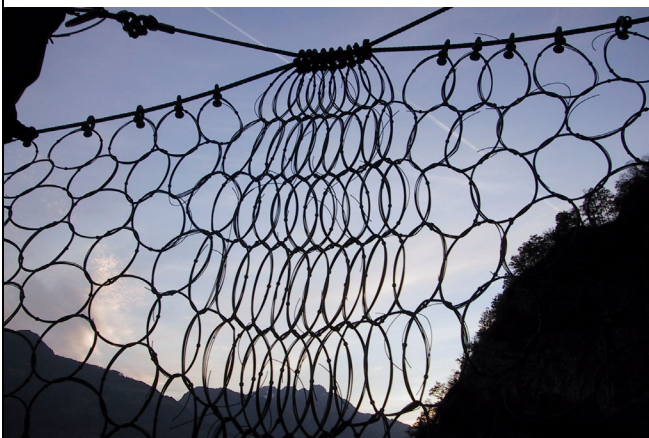
Figure 3. Rockfall protection system after dynamic field test. Note the concentration of the ring net at the position of the maximum cable sag.
