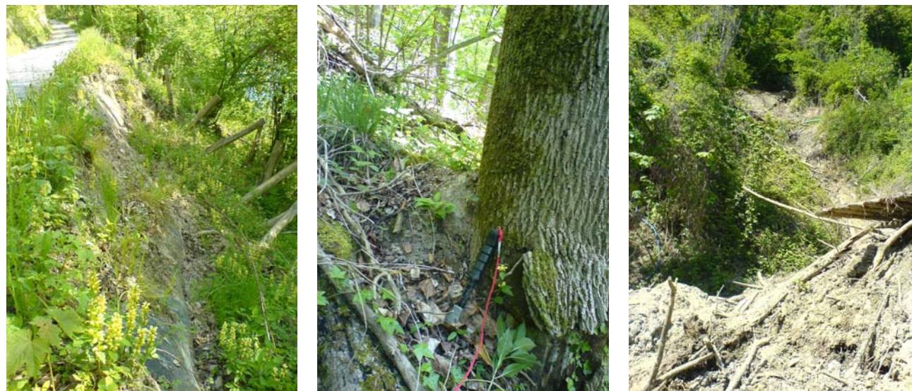
Figure 3: Slide near street, debris flow deposition on tree, debris flow destroyed fence
