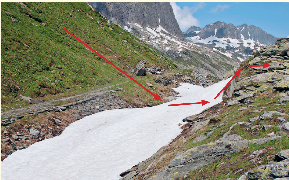
Snow deposits in the Russengraben on 15 July 2013. Just outside the frame of the picture on the right is where the top station of the Nättschen-Gütsch cableway will be built.
