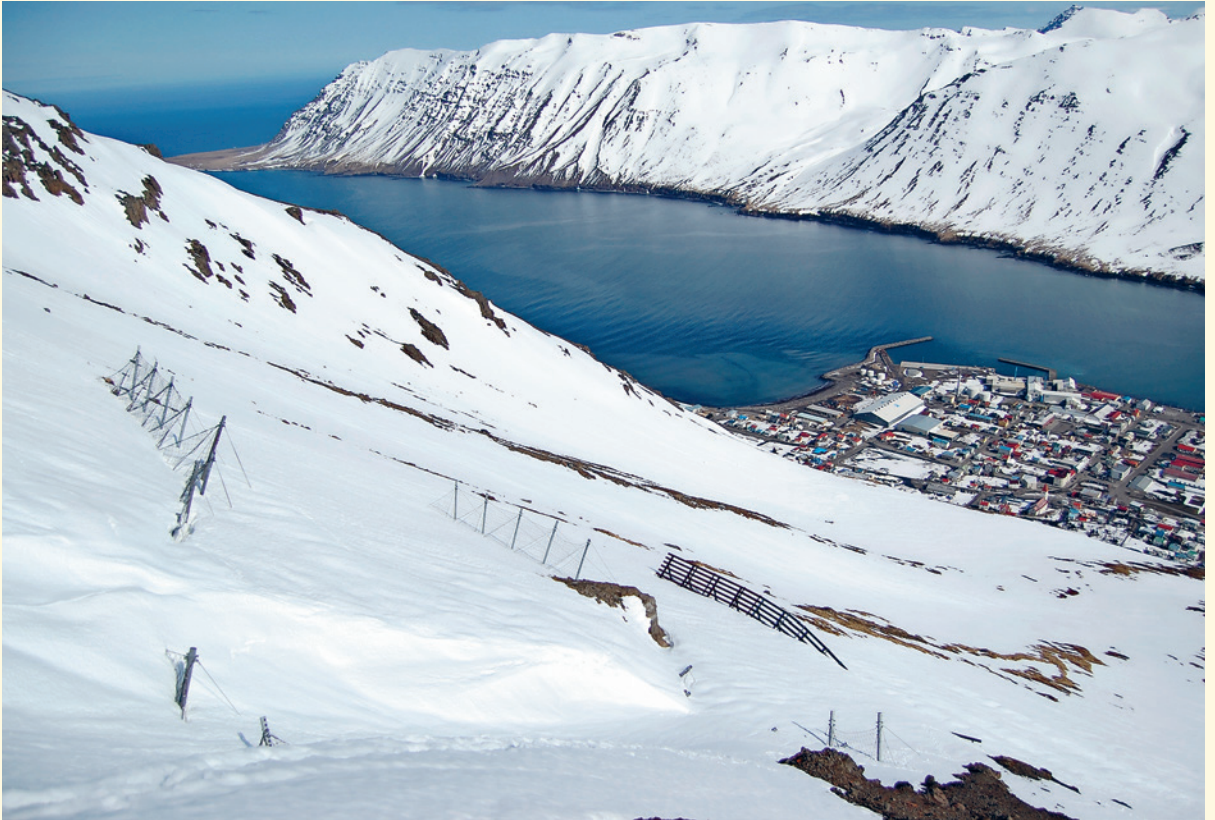
These test installations above Siglufjörður were used to find out which types of structure are suitable for Icelandic conditions. The snow in the foreground is more than 8 metres deep.
